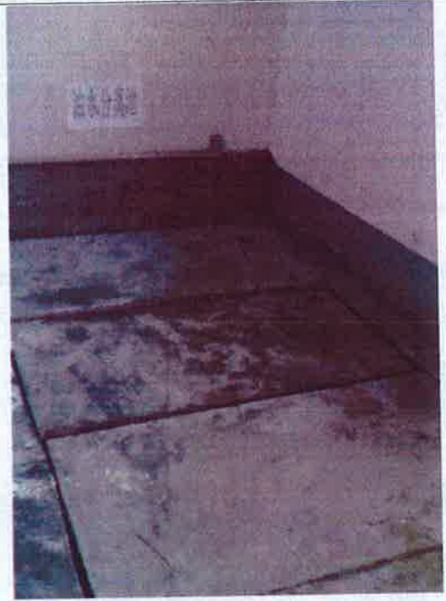
车间隔油池 (0.2m 3 )
